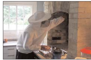
Wasp-Man in action up the kitchen chimney
